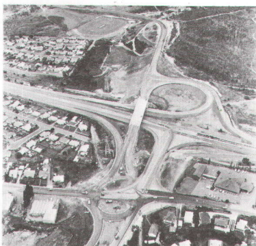
Road construction work on the Tasman Highway at Mornington.
