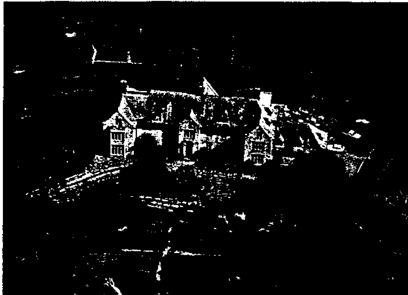
Aerial view of Carrick Hill
