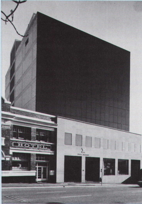
The Macquarie Street, Hobart, headquarters of the Australian Stock Exchange Limited. Photo: Tasmaphotographics
