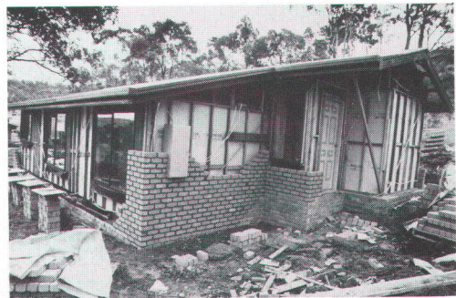
New house being constructed.
