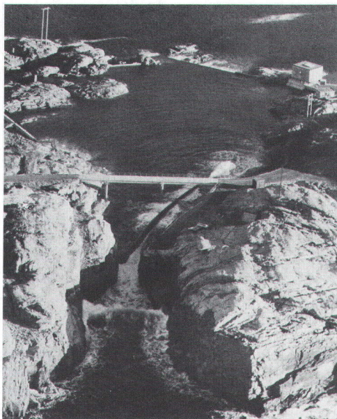
The proposed 1.2MW wave power plant on King Island is similar to this one constructed in Norway.
