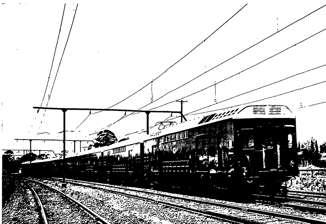
An eight-car all double deck electric train.
