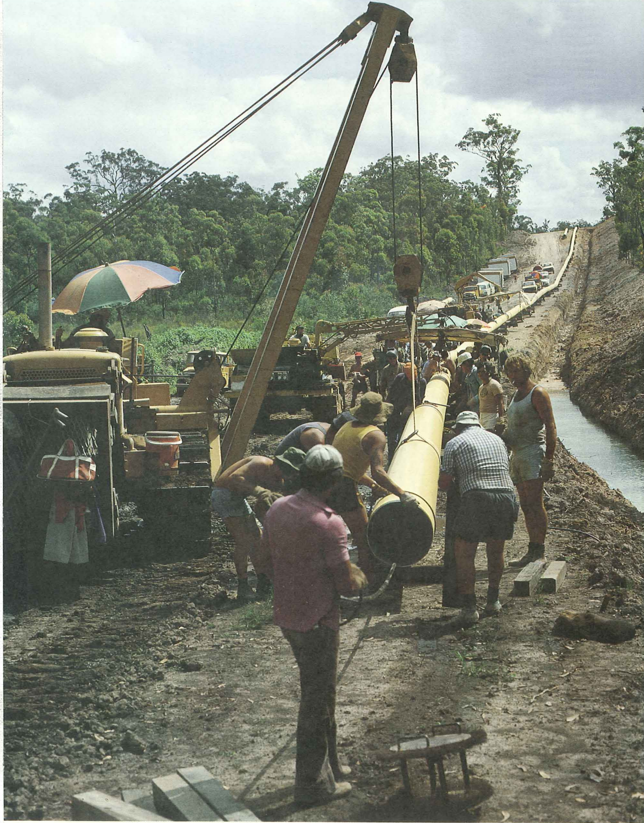
Welding operations on the Newcastle natural gas pipeline.
